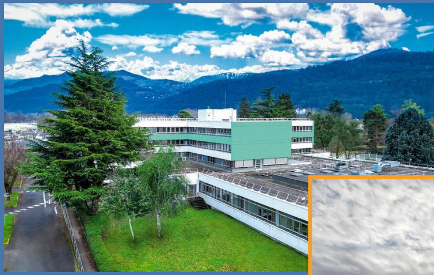
Grenoble, Headquarters & Design center
